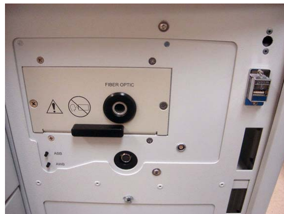
Figure 23 Removing the cabling
